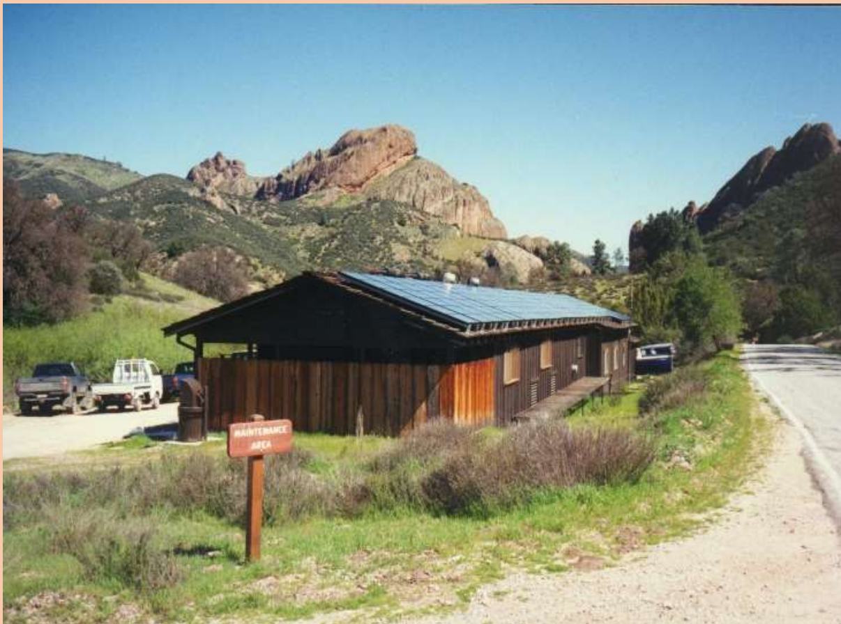
NESI's installation of the original Hybrid PV power system in Pinnacles National Monument, CA
