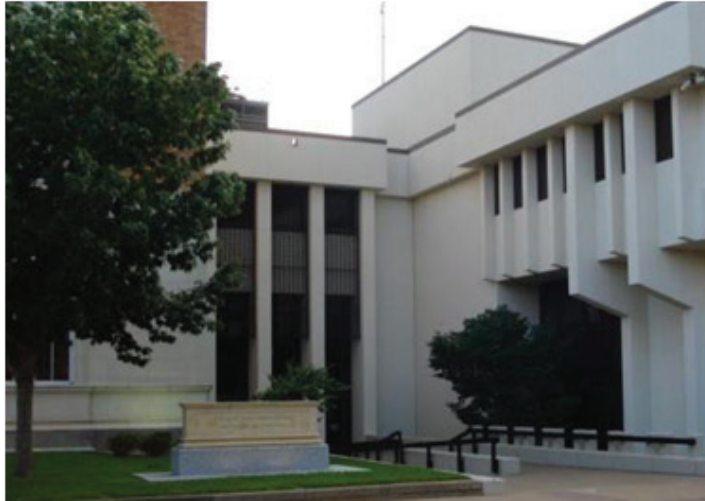
William M. Steger Federal Building & District Court, Tyler, Texas
