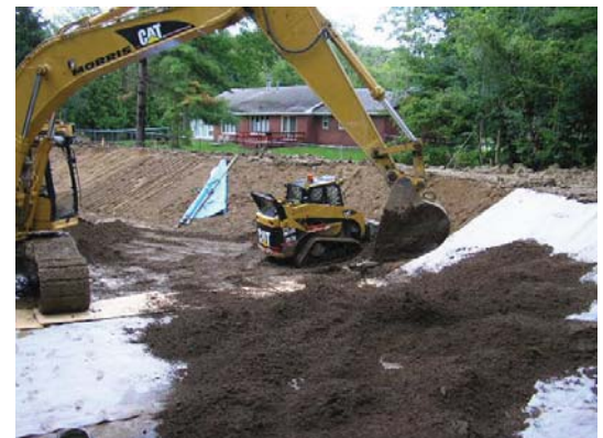
Stormwater Basin Construction
