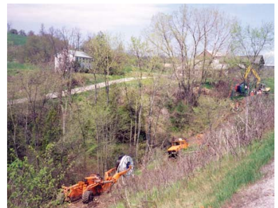
MFS Fiber Optic Cable Installation (cable plows)
