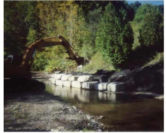
Gas Line Stream Stabilization
