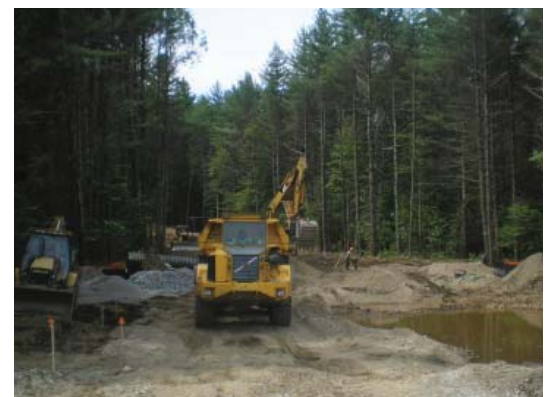
Stormwater Basin Construction
