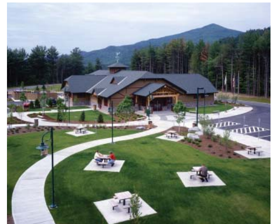
Rehabilitation of Two Rest Areas, NYS Route I-87
