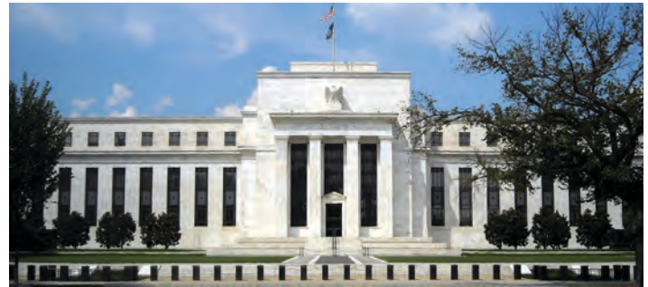
The Marriner S. Eccles Federal Reserve Board Building in Washington, D.C.
