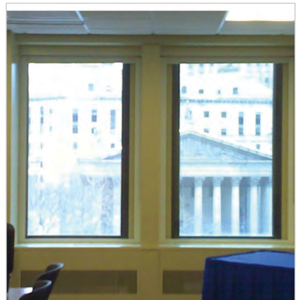
This image shows the existing window (left) beside the installed Thermolite RetroWAL Gold window.
