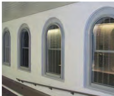
THERMOLITE WINDOWS INSTALLED IN YATES BUILDING
