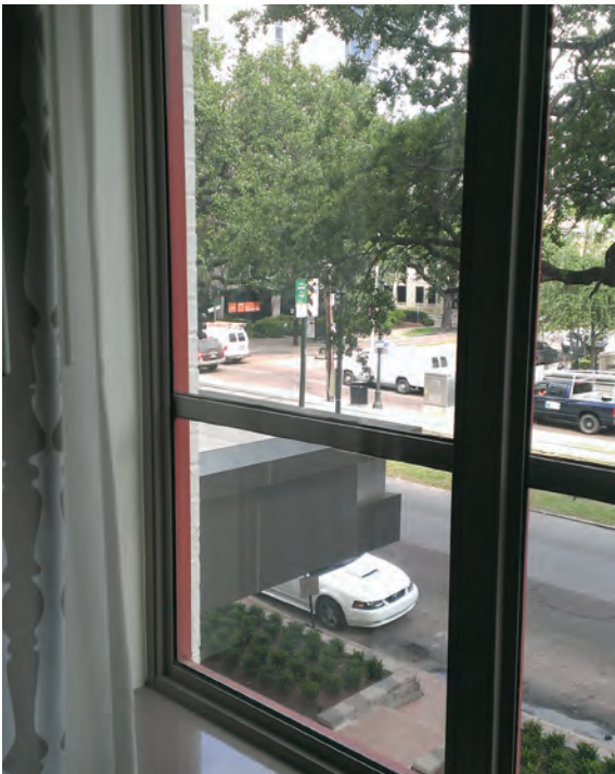
An interior view of a Thermolite blast mitigation window installed at Hotel Indigo.
