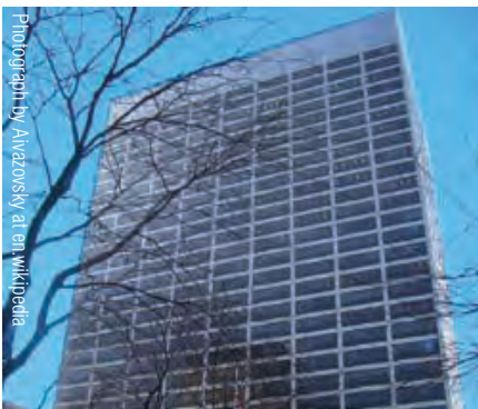
CELEBREZZE FEDERAL BUILDING, CLEVELAND, OH
